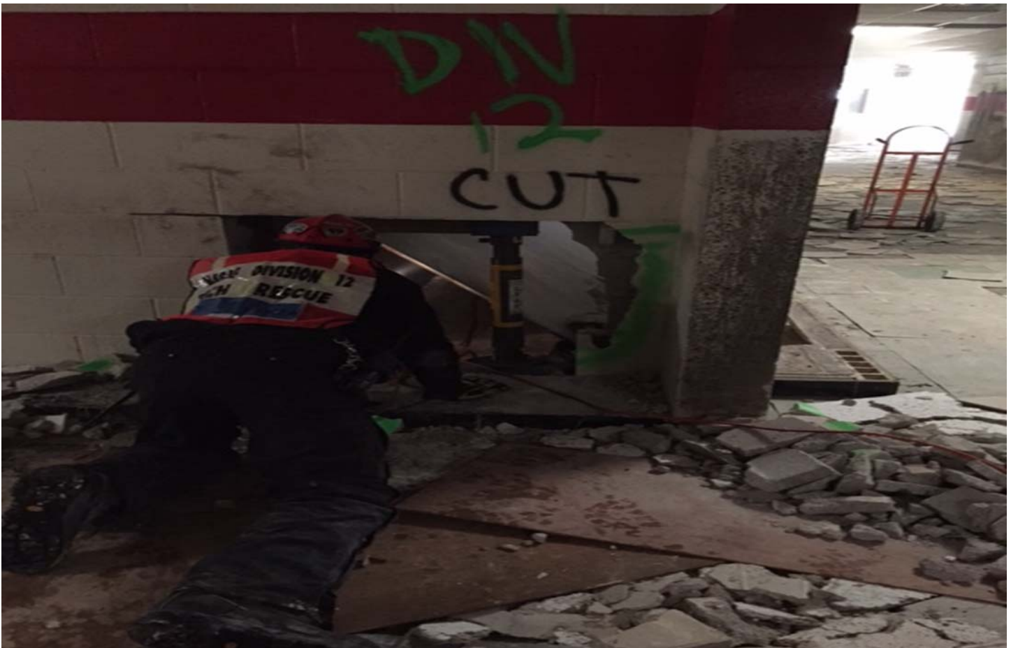
The above picture shows a block wall breach and stabilization with the newly purchased Paratech struts.
