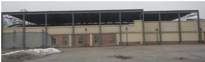
Construction of building exoskeleton to protect bow string roof
