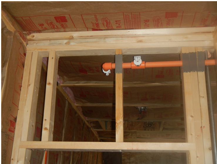
Residential Sprinkler System - Enclave Subdivision
